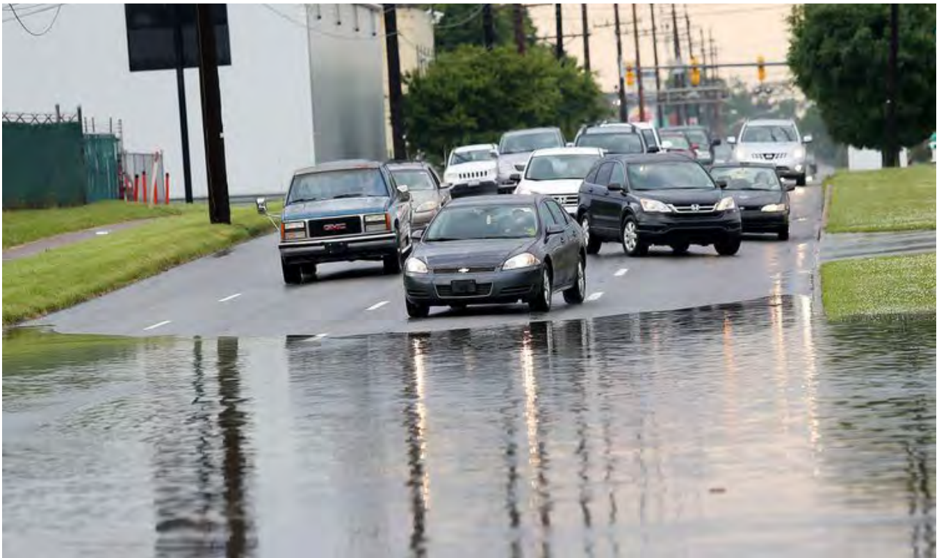
Figure 8: Flooding in the City of Huntington. Photo credit: Chris Chiles, WV Region 2 Planning & Development Council
