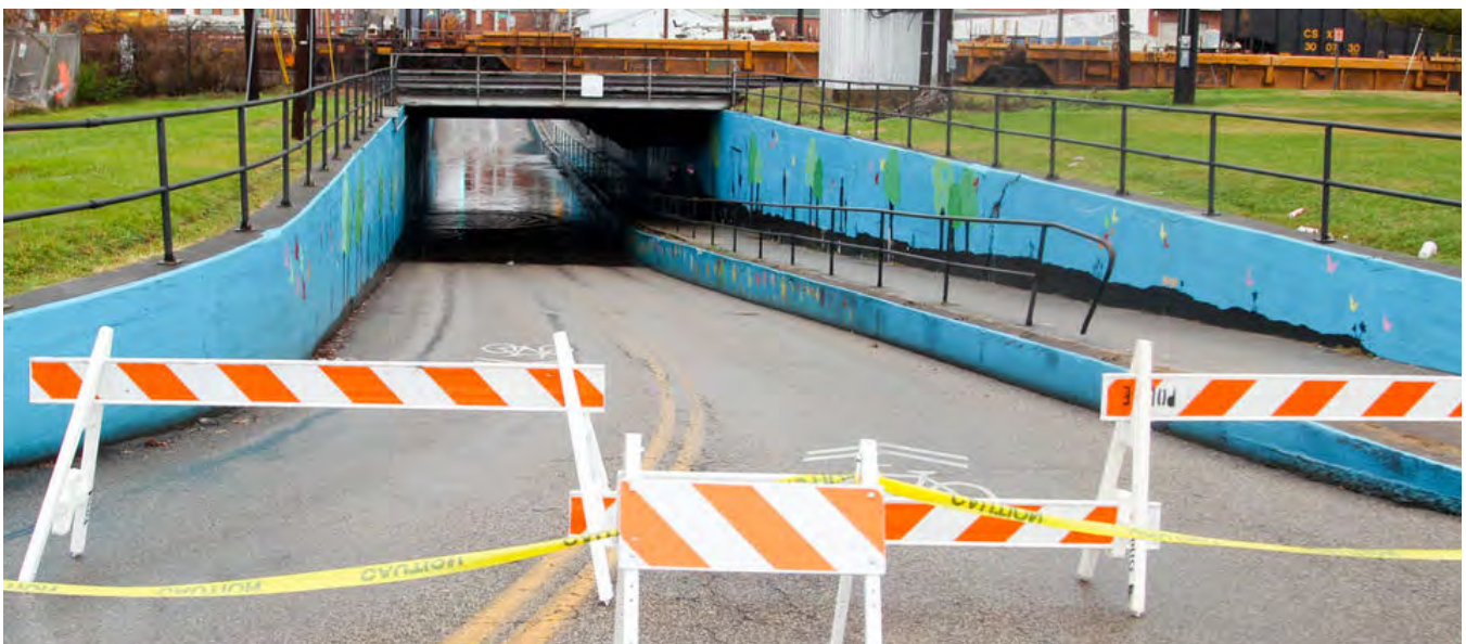
Figure 4: Localized flooding at railway underpasses impacts traffic movement in the City of Huntington. Photo credit: Sherry Wilkins, HSU
